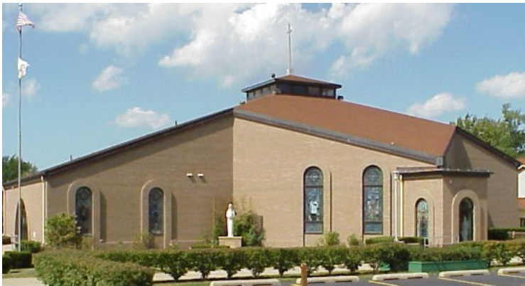
Saint Lawrence Church 180 East State Street Albion, Pa. 16401 Founded 1914
