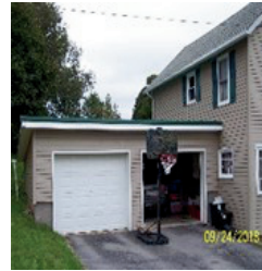
(L) After-insulation fixed.
